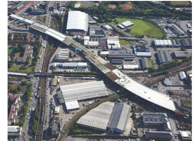
M74 - Port Eglinton Viaduct
