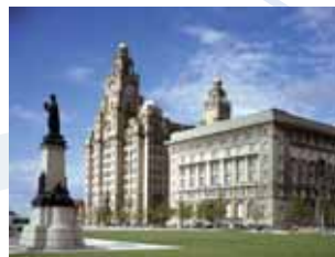
Exterior of Liver Building, Liverpool
